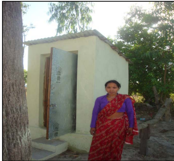
Fig 1 HH Latrine constructed in Shibnagar TP. Source: ADB, Nepal: Second Small Towns Water Supply and Sanitation Services Project.
